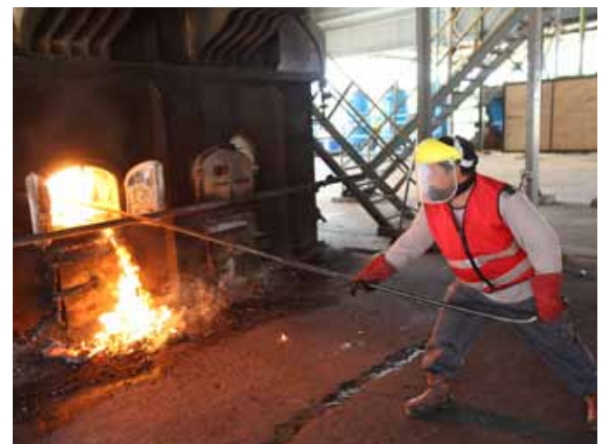
Boiler handler at PTNJL
